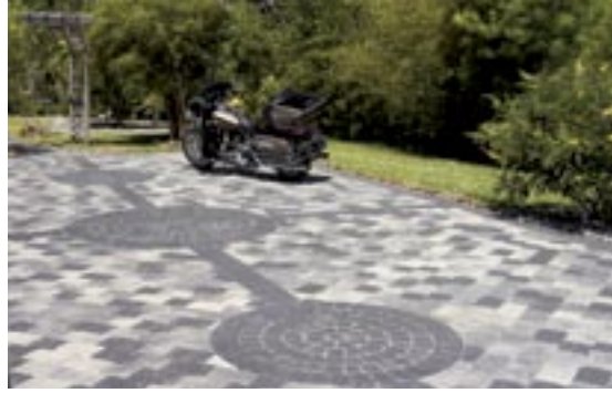
Driveway using Appian-Stone® combo with Classico® circles inset for a dramatic look.
